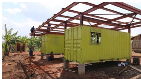
Kyamugarura mini-grid during construction shipping container mounted superstructure
